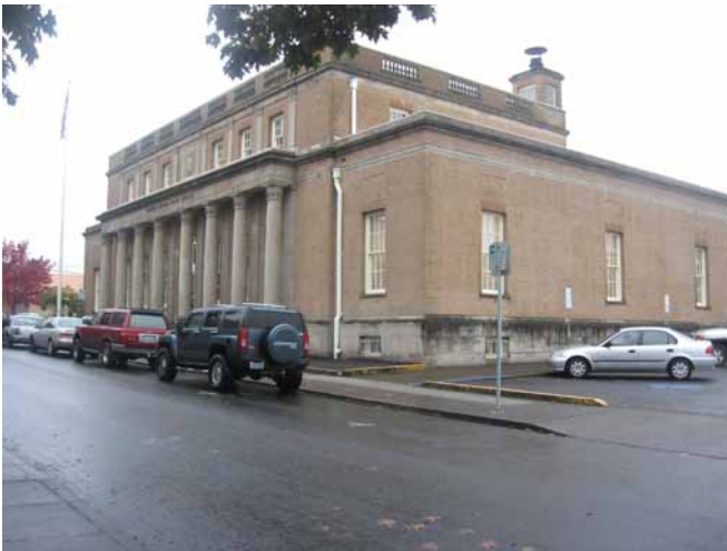
Existing Building (Post Office) North of Site
