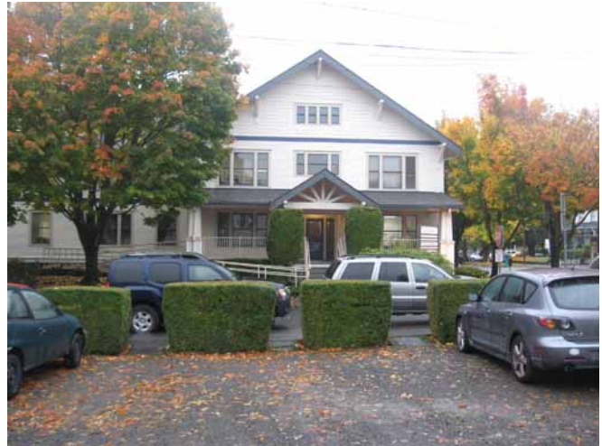
Existing Building West of Site
